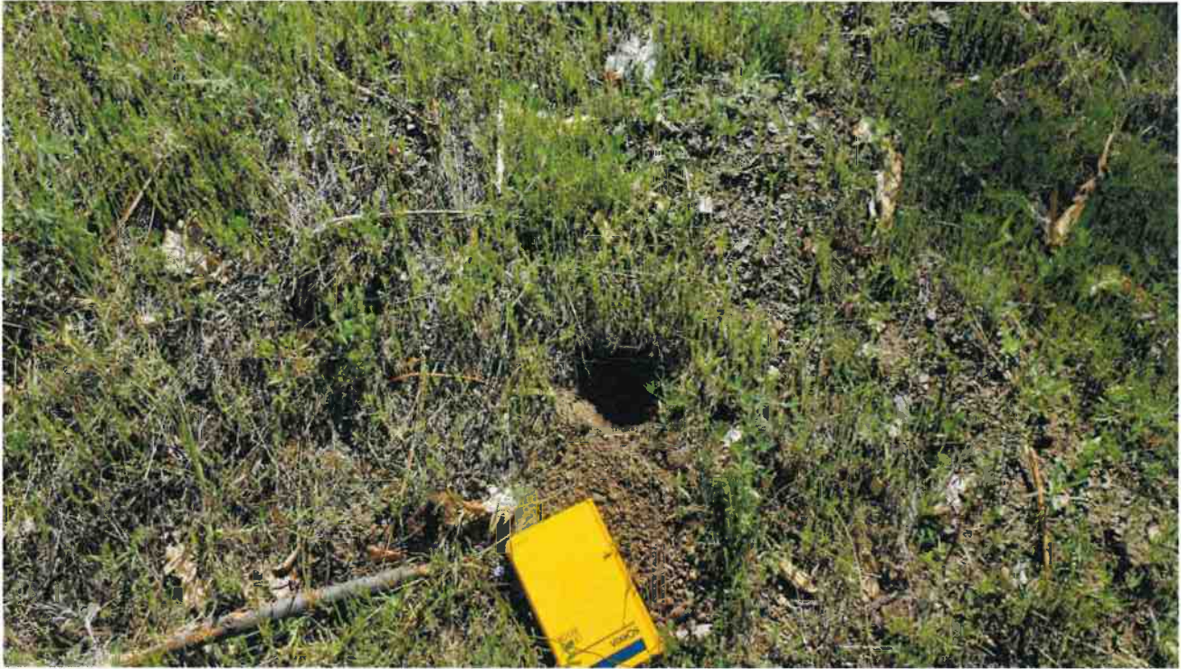
4. View of large rodent burrow at downstream right groin.
