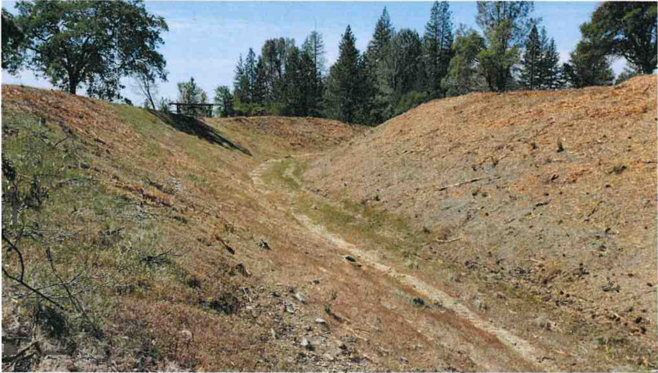
6. View of downstream spillway channel.
