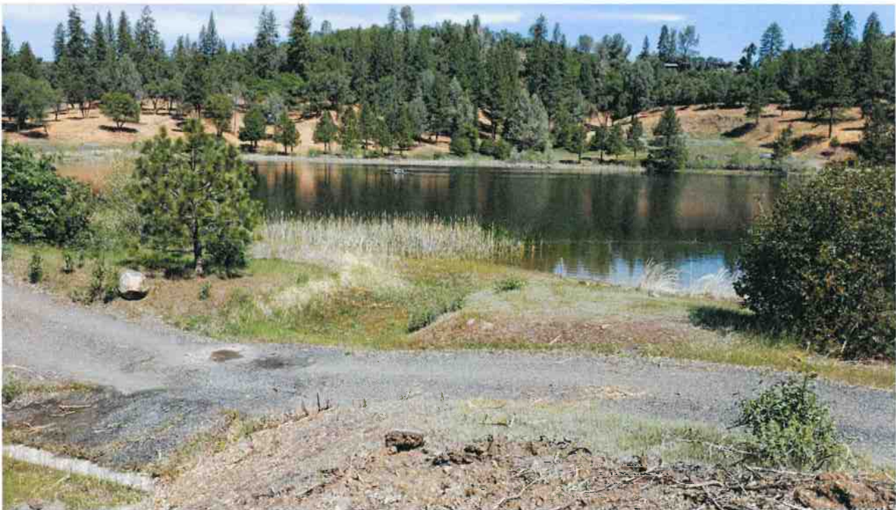
5. View of spillway approach and control.
